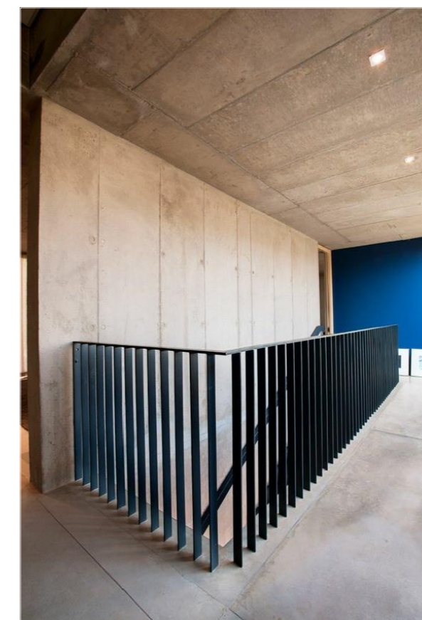
5 Black mild steel balustrade
